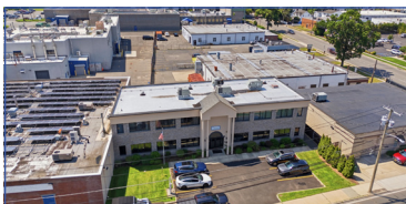
219 Dixon Avenue 8,000 SF Administrative
