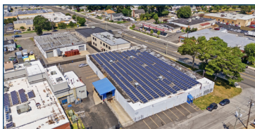
225 Dixon Avenue 21,000 SF Warehouse & Quality Control
