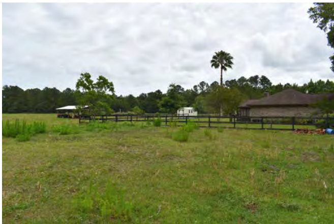
9. 5670 residence-auxiliary building and barn
