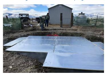
Figure 50: Insulation of hot spring.
