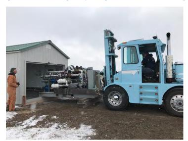
Figure 52: Off-loading and placing DER unit inside building.
