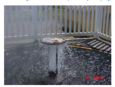
Figure 59: Artesian geothermal well at Surprise Valley Hot Springs resort.
