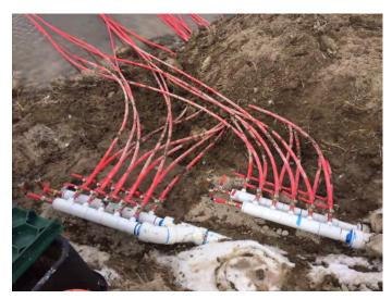
Figure 46: Installation of cold water loops.
