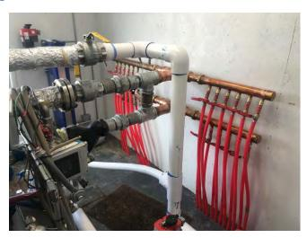
Figure 45: Cold water manifolds.
