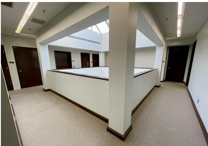
2nd floor Atrium
