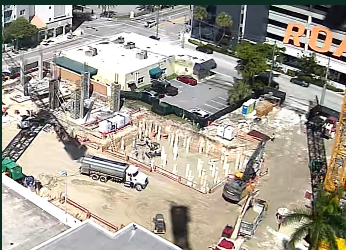
Construction progress — tower crane on site, September 2026.
