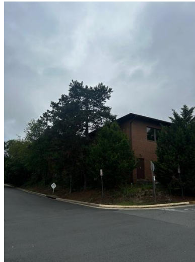
Back of building
