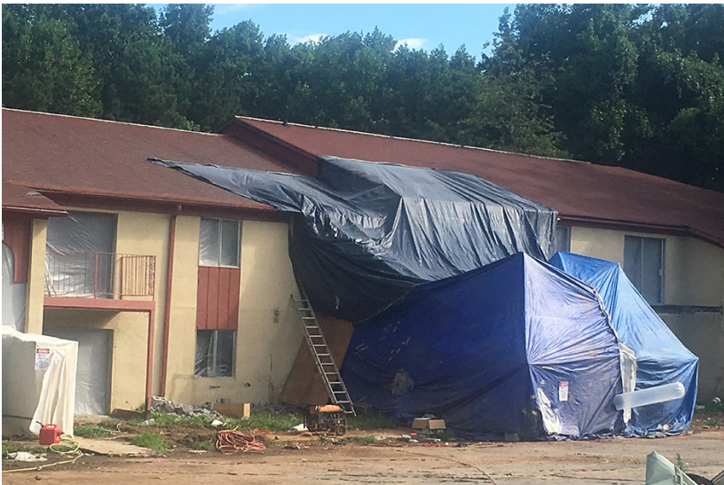
Photo of Property during demolition – Summer 2016
