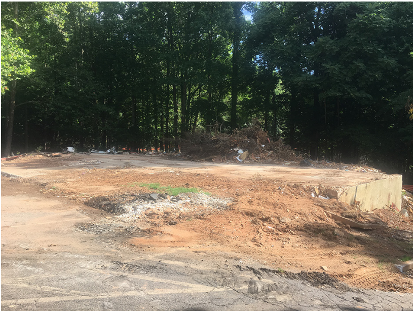
Photo of Property during demolition – Summer 2016
