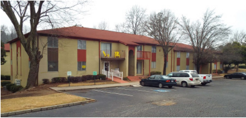
Photo before demolition – Summer, 2016
