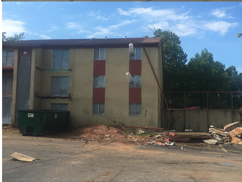
Photo of Property during demolition – Summer 2016
