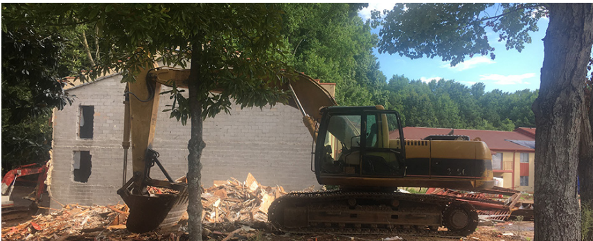
Photo of Property during demolition – Summer, 2016
