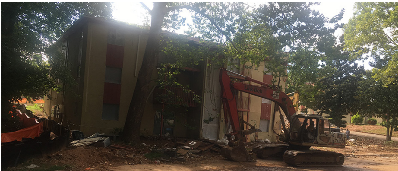
Photo of Property during demolition – Summer 2016
