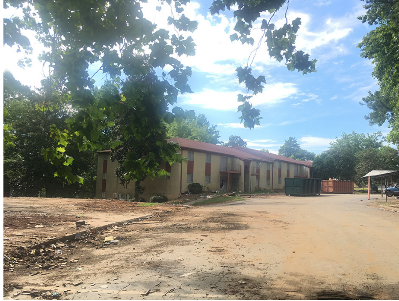
Photo of Property during demolition – Summer 2016
