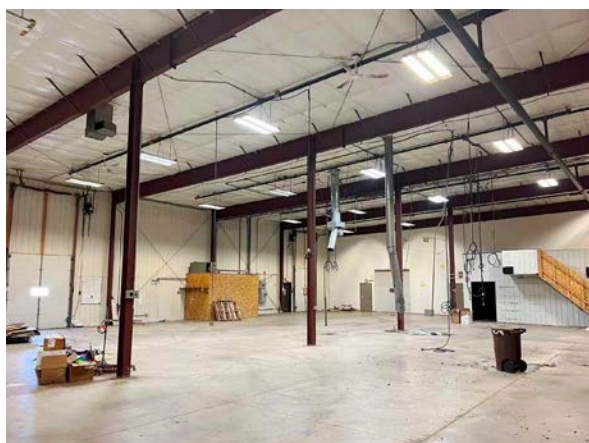
West Section: Warehouse
