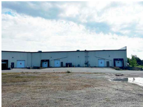
Back Side of Building/Overhead Doors
