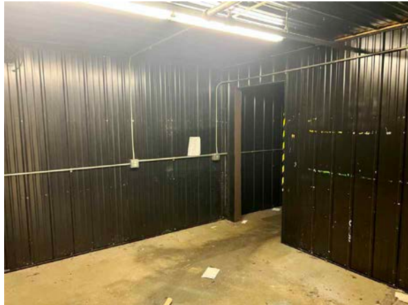
West Section: Paint Room
