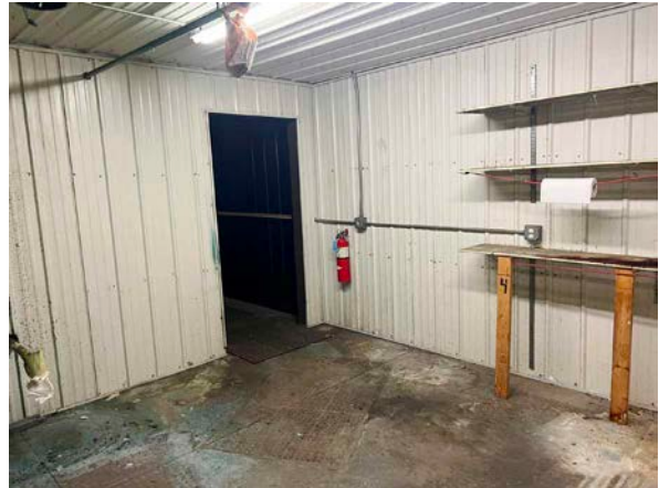
West Section: Paint Room
