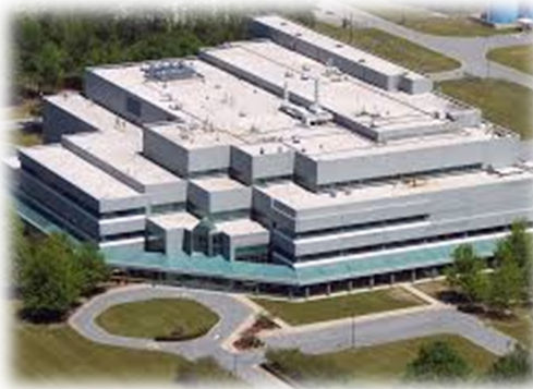
Large Industrial Facilities
