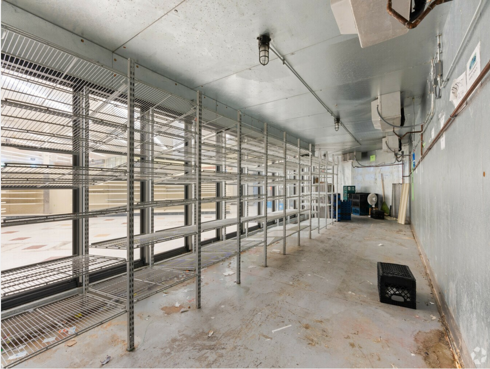
Rear of Refrigerator Room
