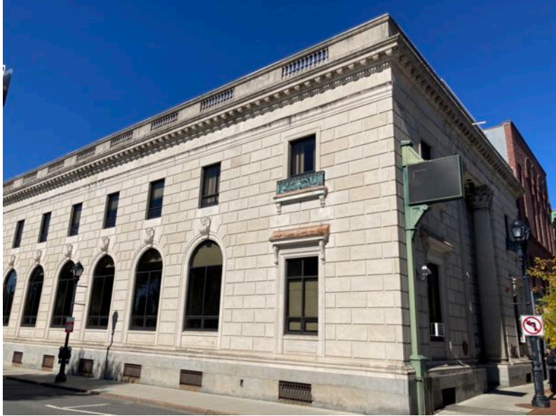
74 Concord St - Exterior
