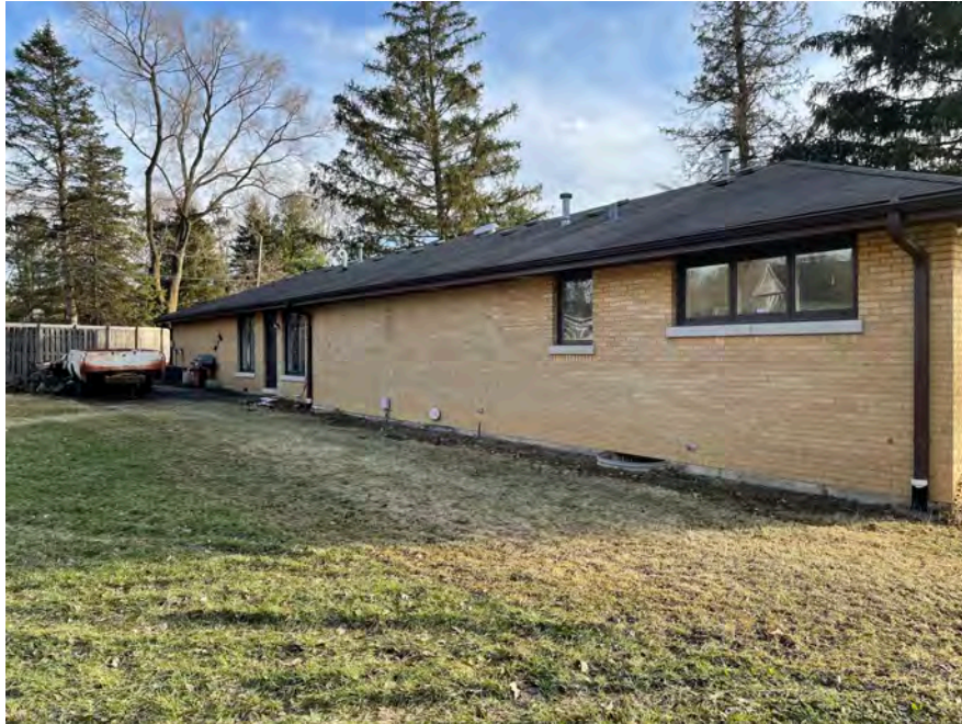
North Side of Main Building
