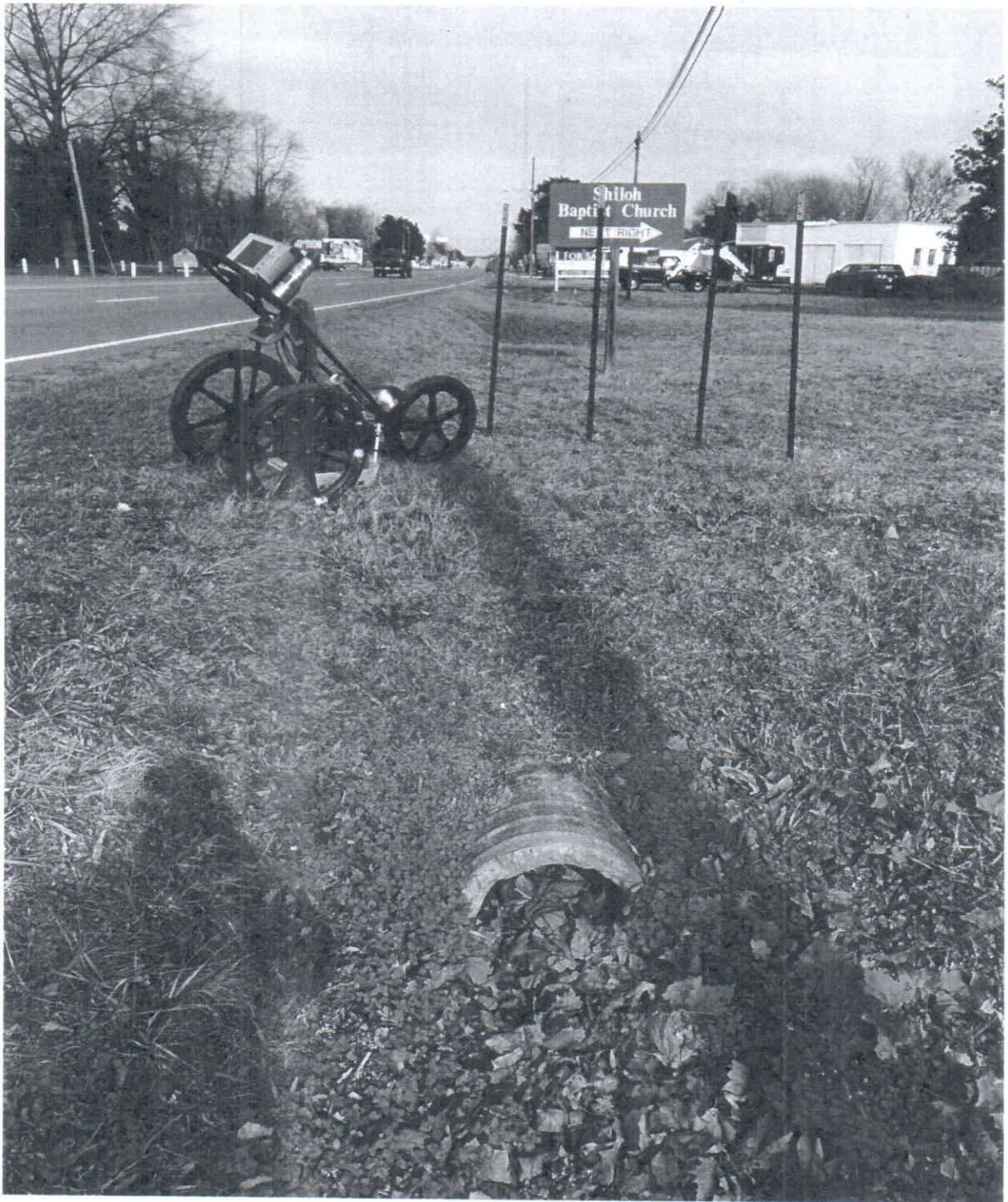
This image shows the pipe running in the ditch alongside the road which was able to be located on the radar.
