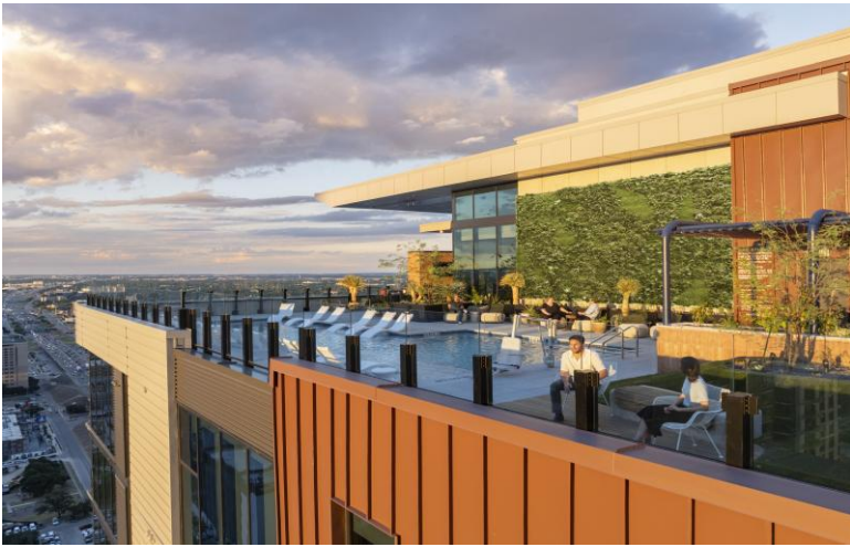
Rooftop Pool — Top-Floor Amenity Deck
