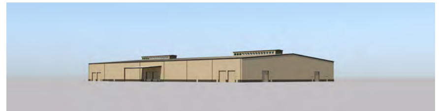
CORNER VIEWS - BLDG K North East - Top | South East - Bottom
