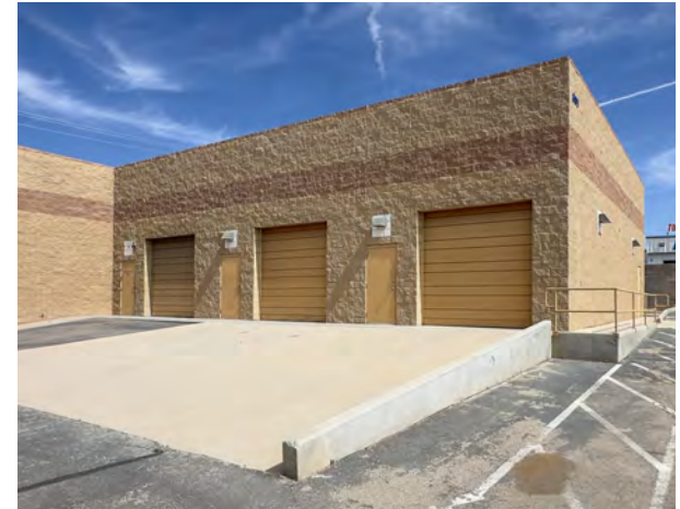
Concrete drive-in ramp for two doors
