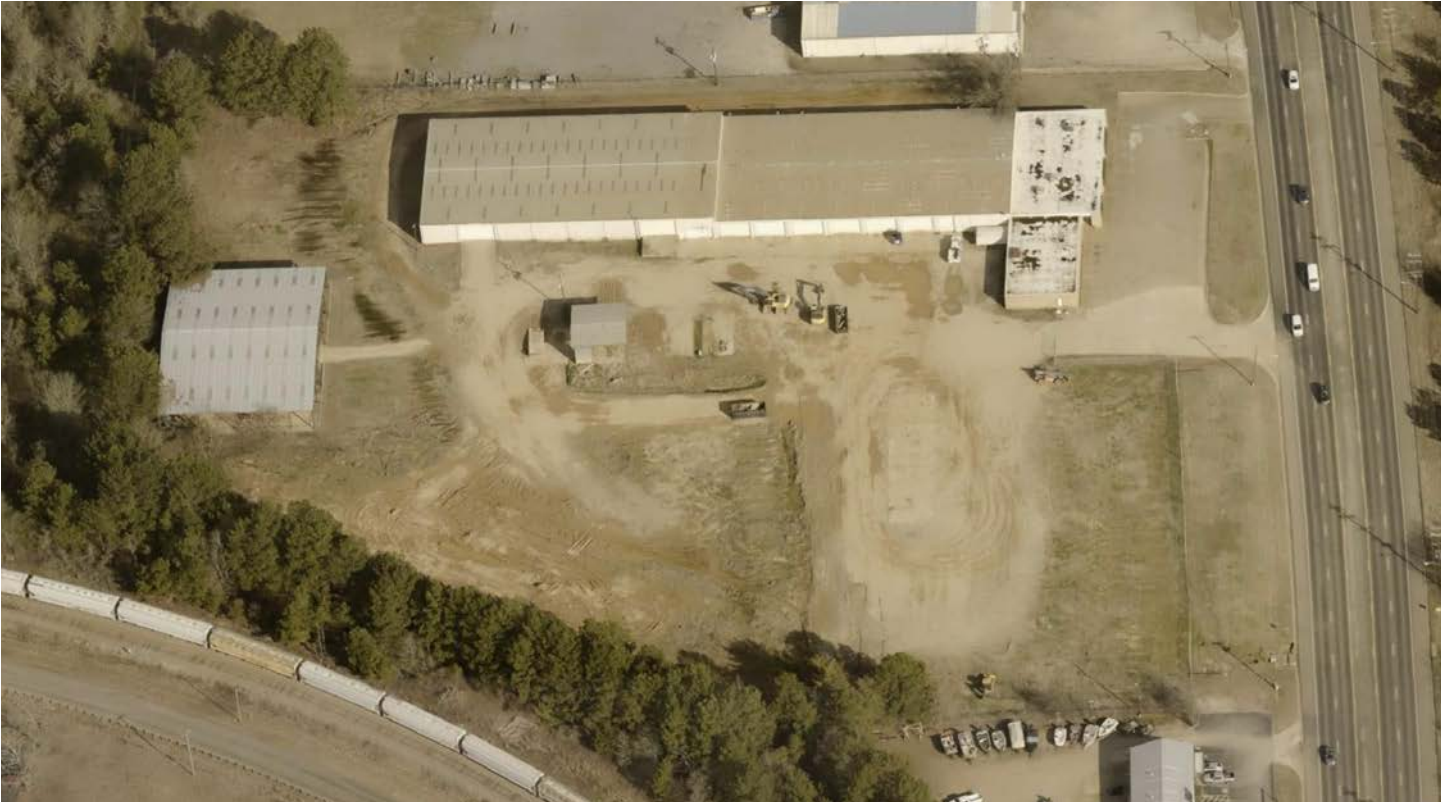
Aerial image of south side of building.
