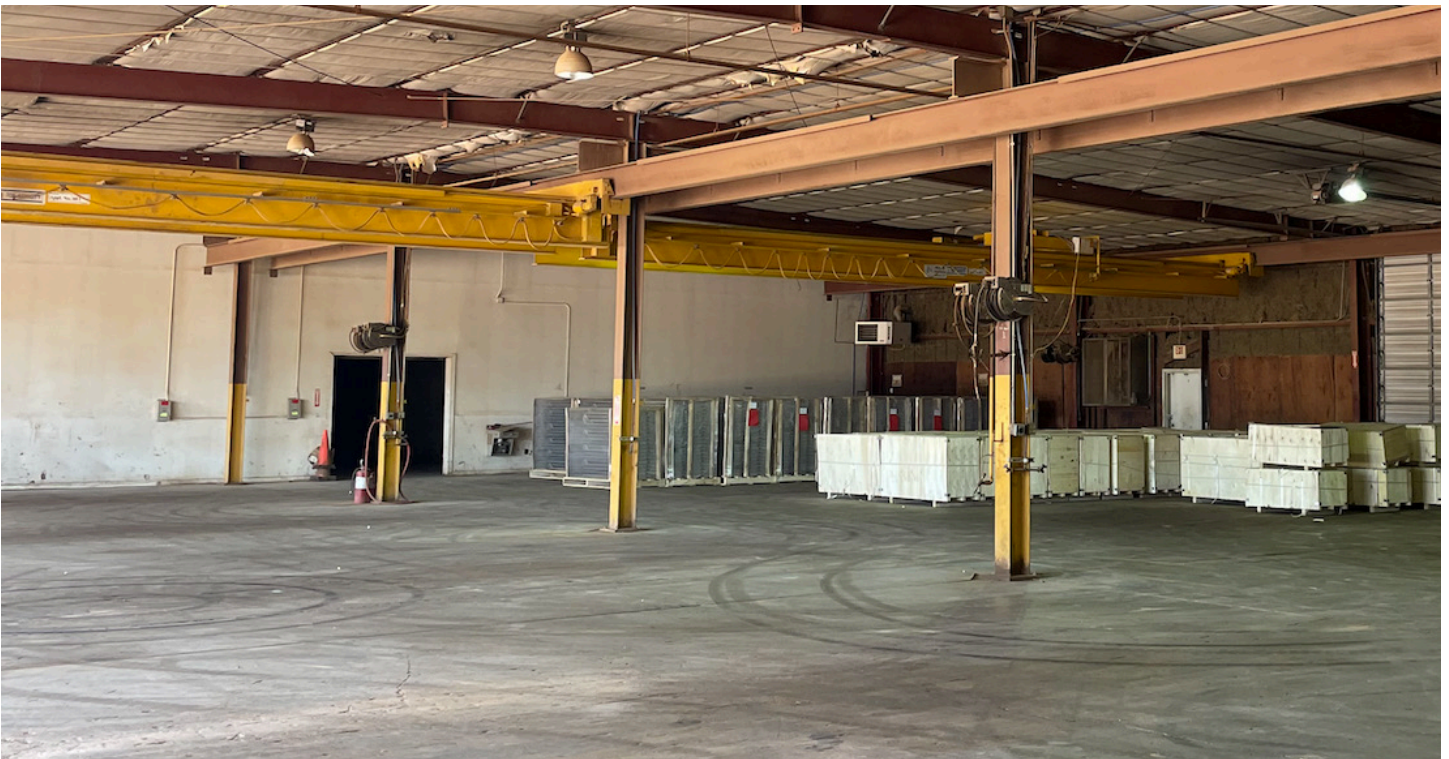
Main shop area looking in towards the northwest corner.
