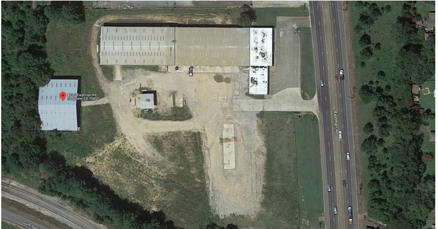
Aerial view of site
