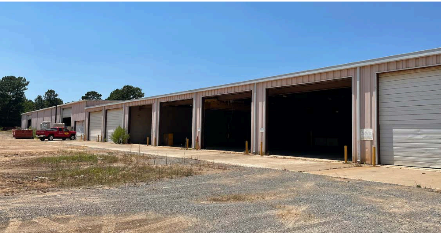
Shop doors along south side of building.
