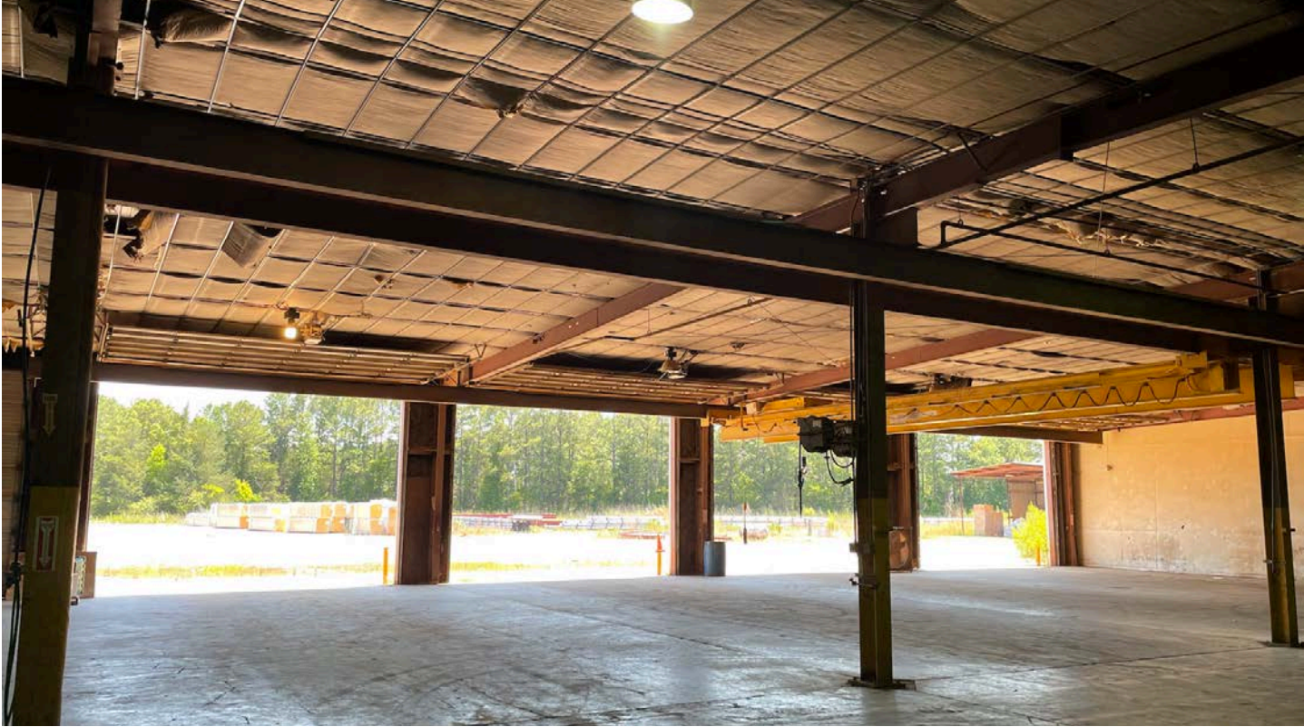
Main shop area looking out towards the southwest corner.
