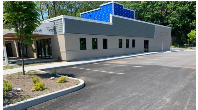
Shell Space Ready for Build Out
