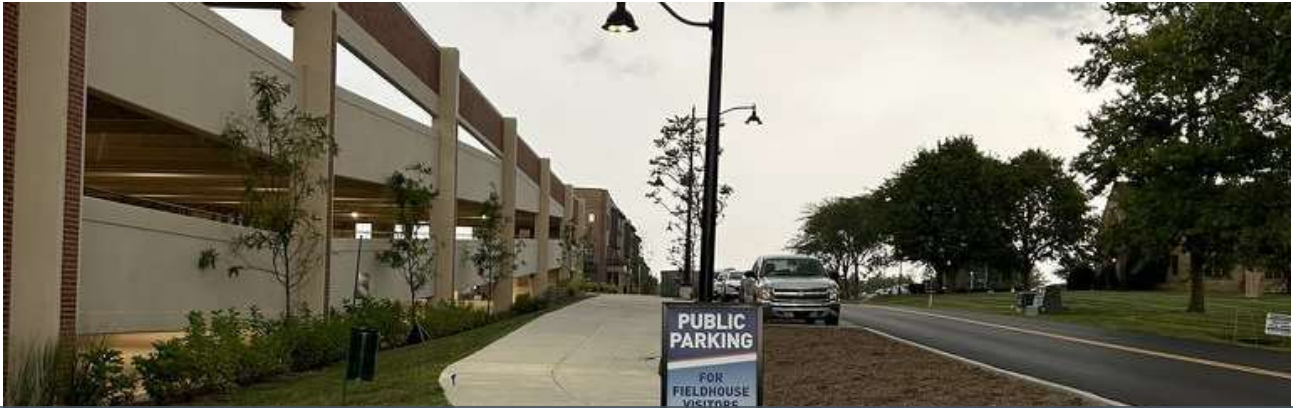
354-Space Parking Garage
