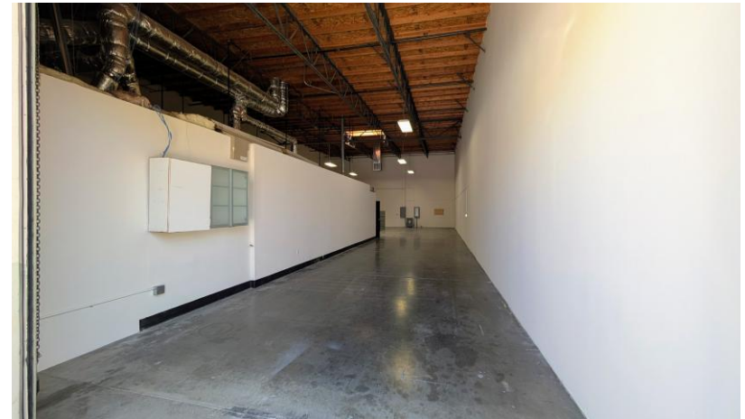
Front-loaded warehouse with power distributed throughout.
