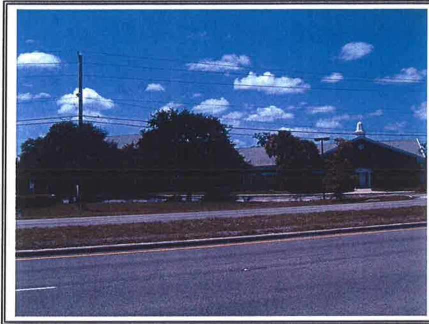
Photo No. 1: View of the Subject Property facing west.
