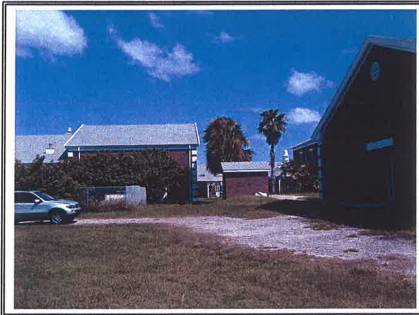
Photo No. 10: Photograph of interior courtyard from the south facing north.
