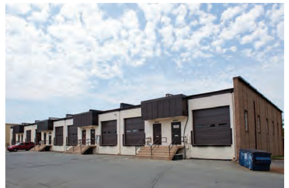
Loading Dock Entrances
