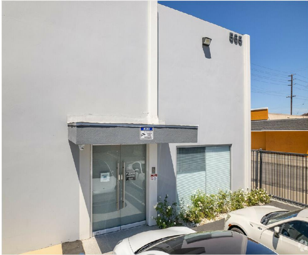
Back Entry from Parking Lot
