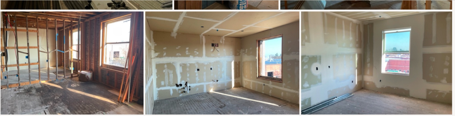
BUILDING INTERIOR · RENOVATION IN PROGRESS
