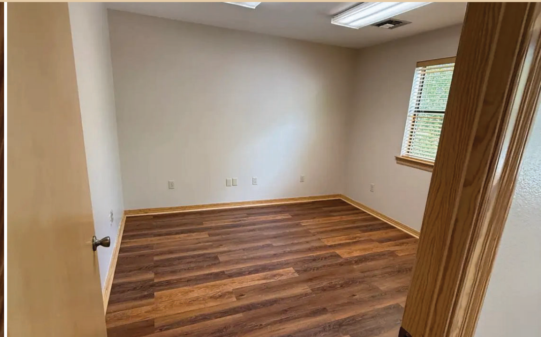
INTERIOR OFFICE DETAIL
