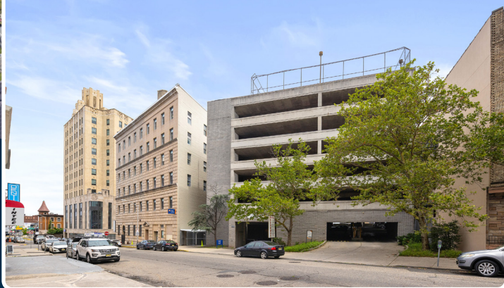
PARKING DECK ACCESS VIA PROSPECT ST
