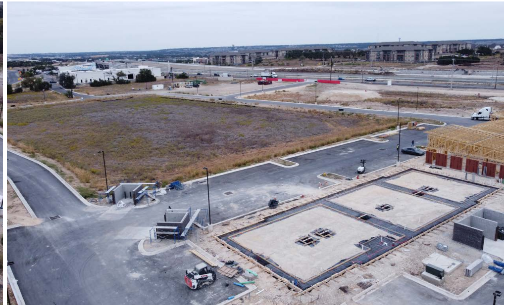
Construction Progress Oct 2024
