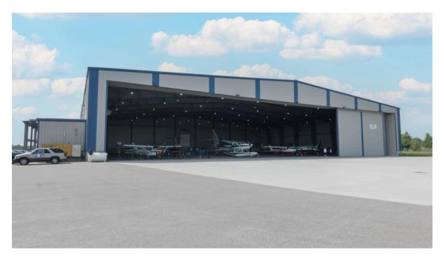
200 feet of heated hangar doors creating open span of up to 150' in width.
