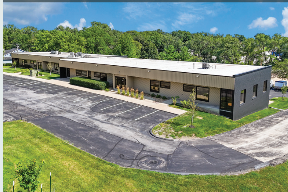
Upper Level - North Side
