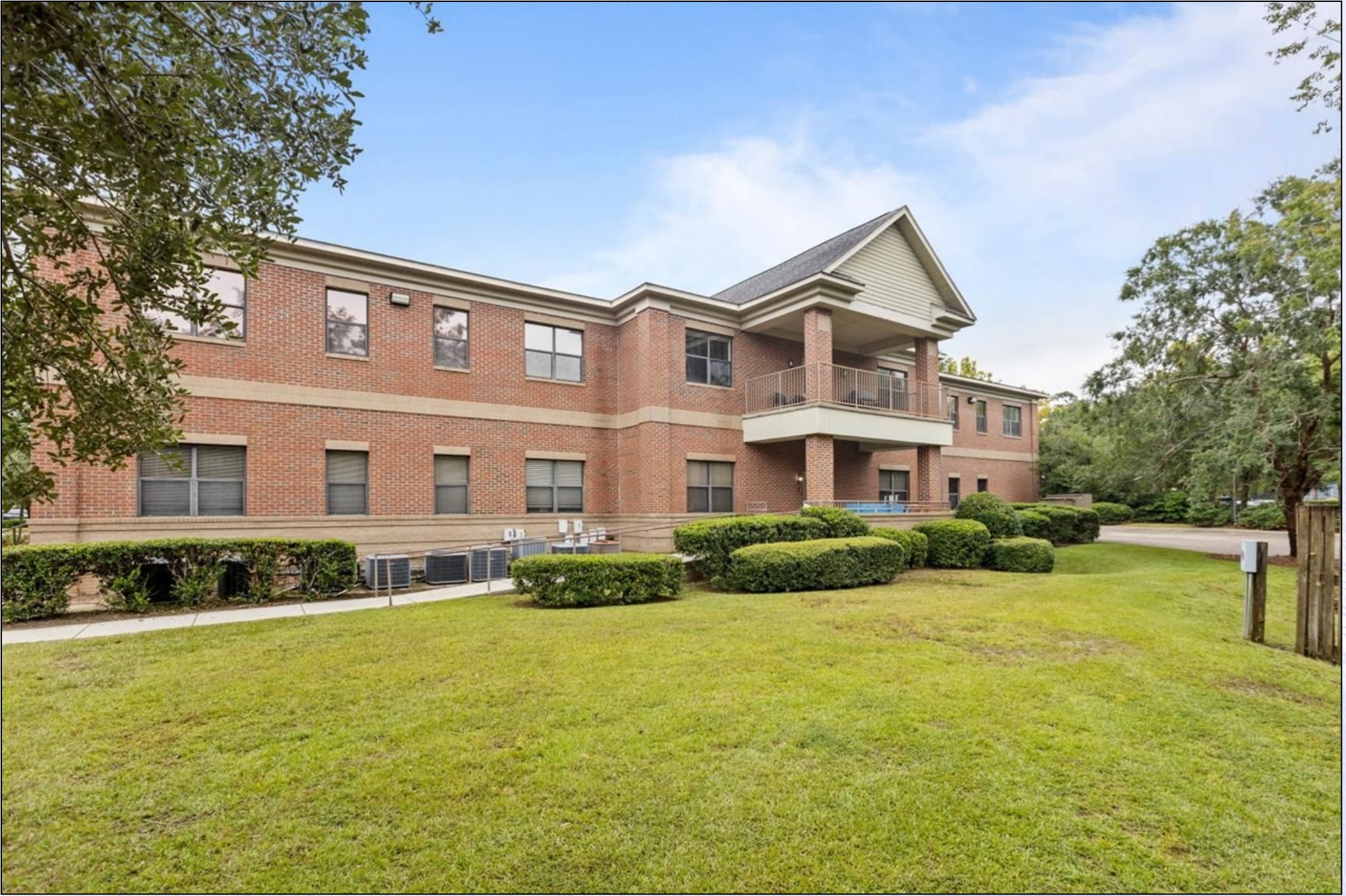
Exterior View Rear (Showing Covered Porches)
