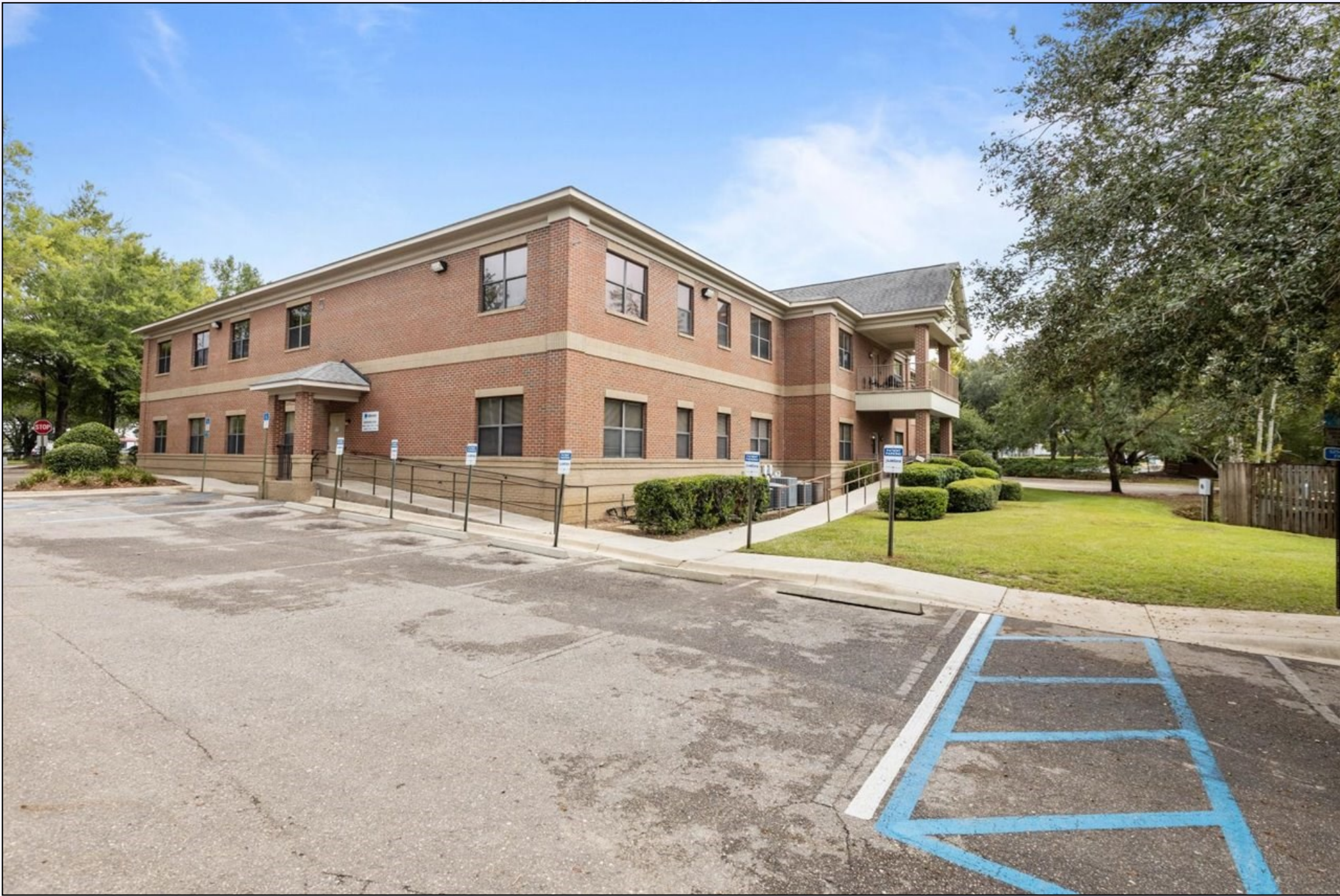
Exterior View (North Side)
