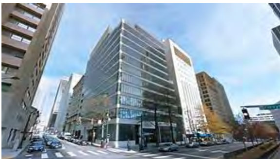
41 Marietta Street Tower
