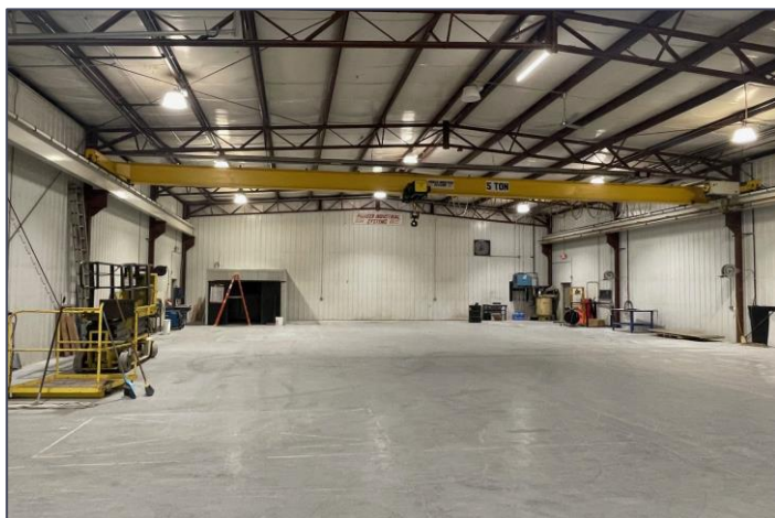
Crane Bay – Built For 10-ton Capacity
