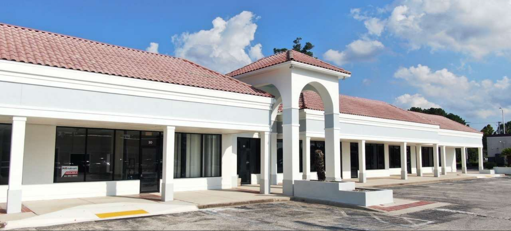
New Facade & Paint
