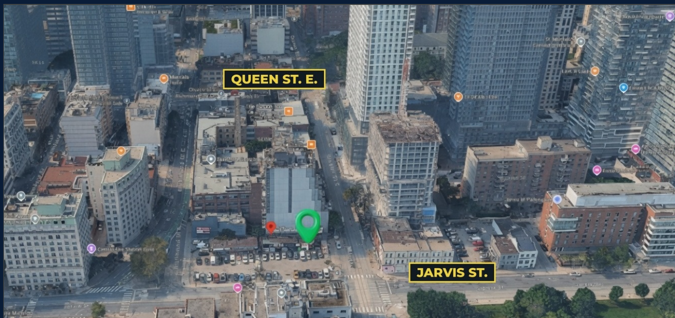
AERIAL · QUEEN STREET EAST AT JARVIS · DOWNTOWN TORONTO EAST
