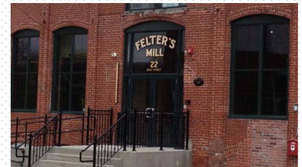
Felter's Mill—mixed commercial development
