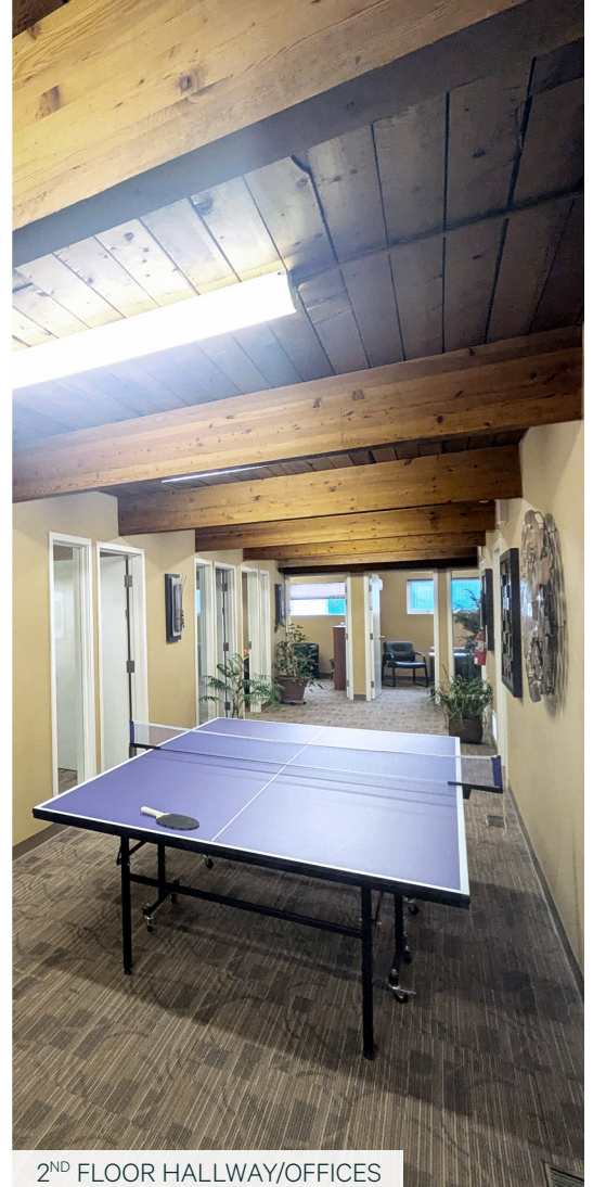
2 ND FLOOR HALLWAY/OFFICES
