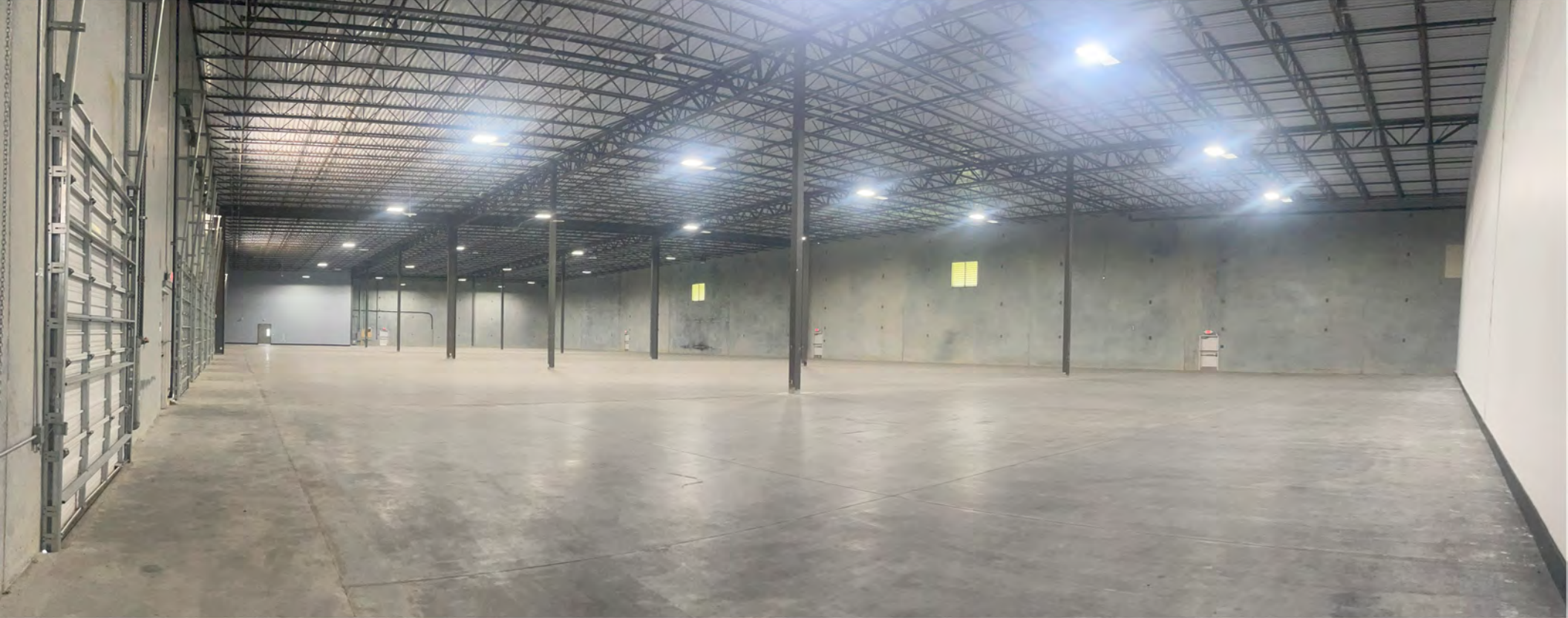
VIEW FROM NW CORNER OF WAREHOUSE
