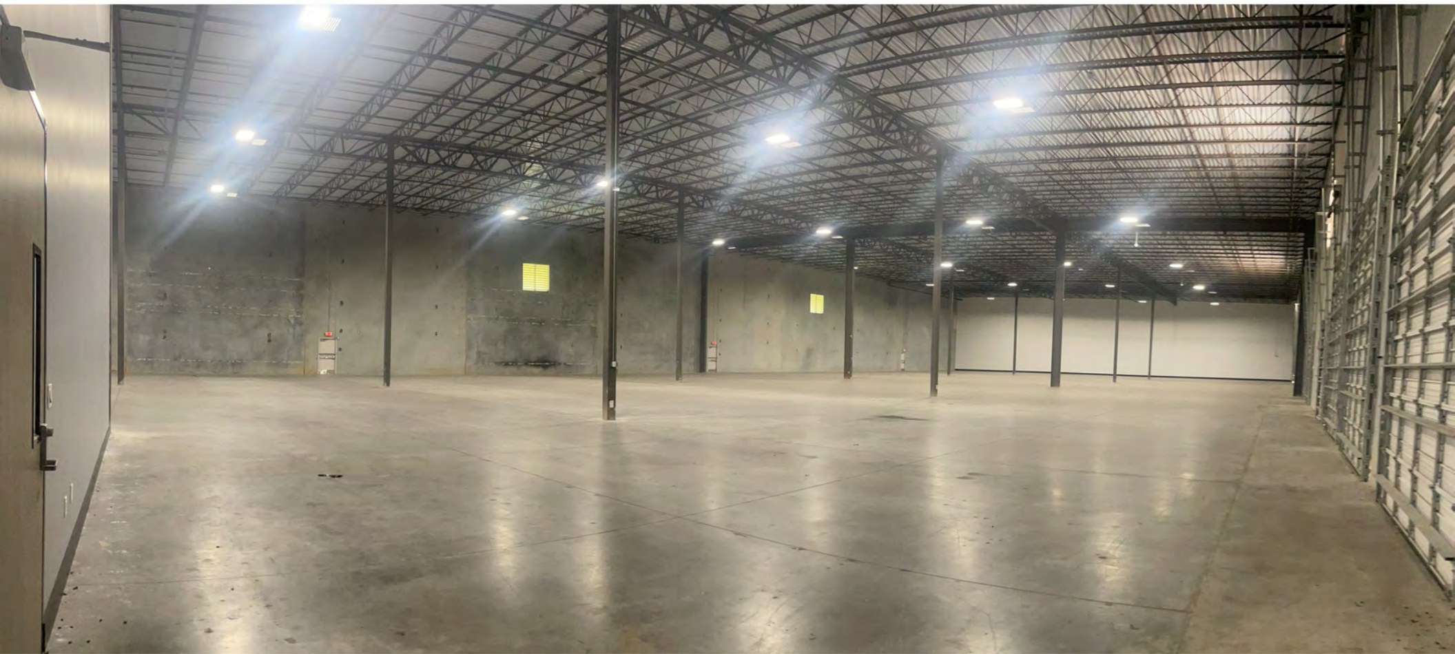
VIEW FROM SW CORNER OF WAREHOUSE
