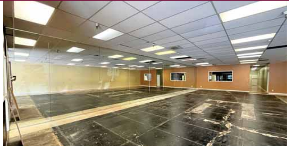
6940 Interior - Former Martial Arts Studio
