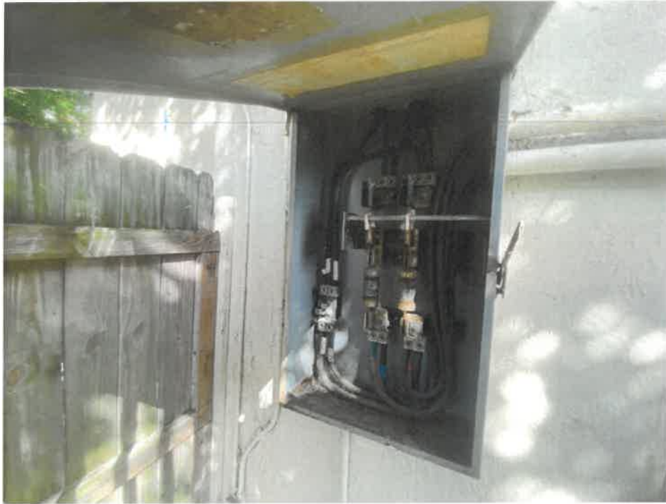
10. View of Grounding of Branch Circuit Equipment
