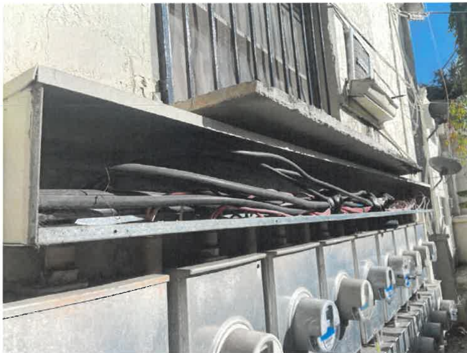
6. View of Electrical Gutters, Wireways
