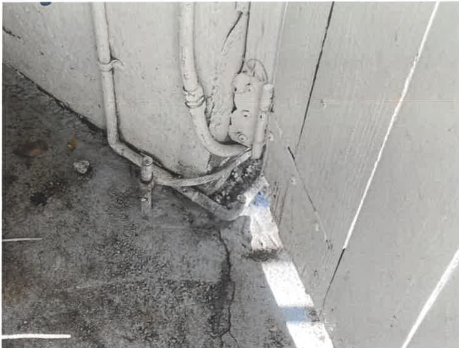
9. View of Grounding of Service
