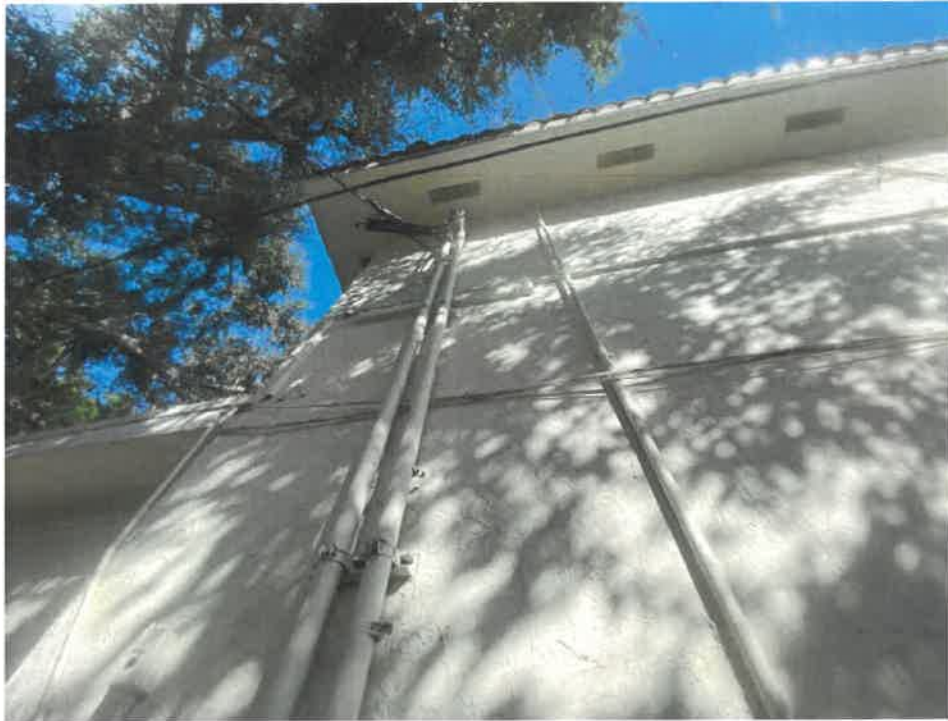
11. View of Service Conduit/Raceways
