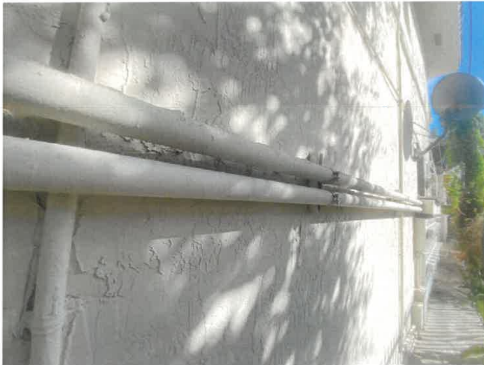
11. View of Service Conduit/Raceways
