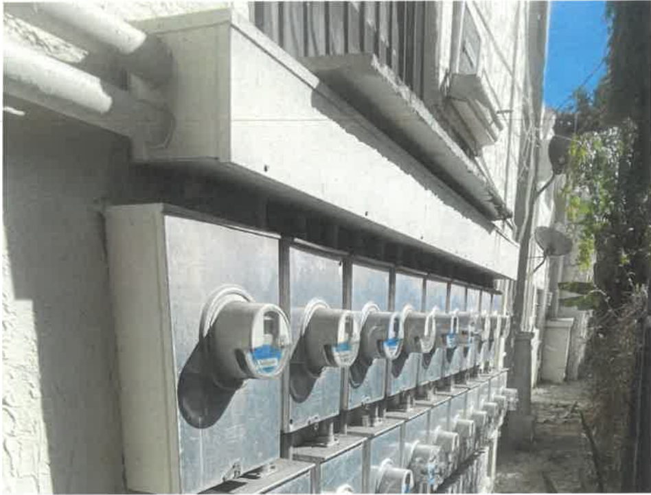
6. View of Electrical Gutters, Wireways
