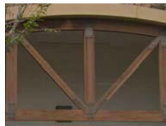
10 WOOD ARCHWAY BROWN TEAK WOOD REF. MATCH EXISTING SHIPPING CENTER REF. MATCH EXISTING SHIPPING CENTER COLOR CUSTOM BROWN SEE 3/A-400
