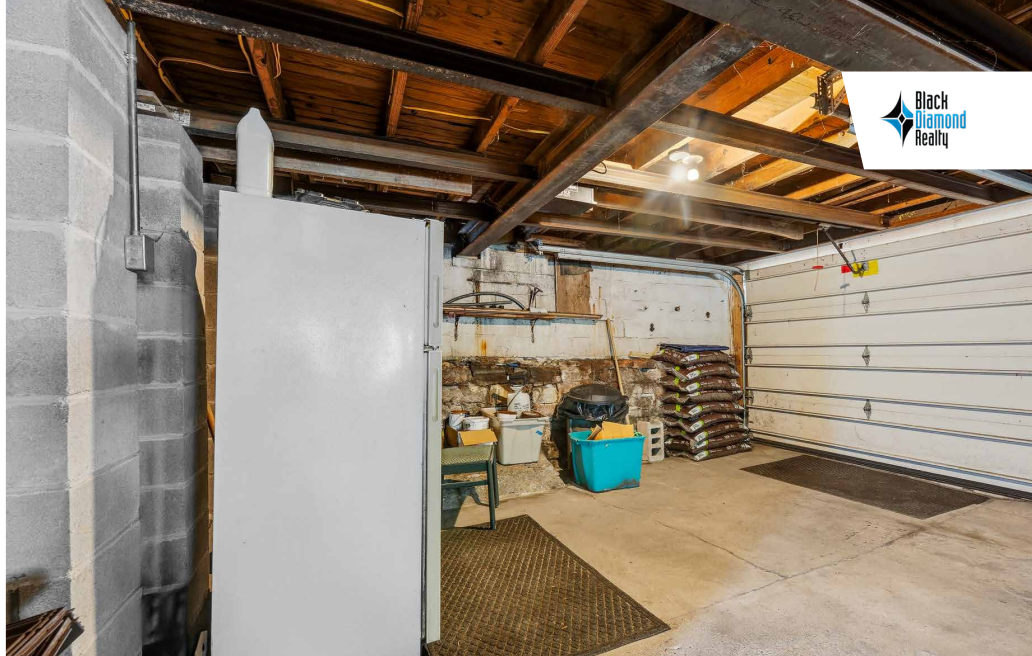
Restaurant Building Basement with Overhead Door.
