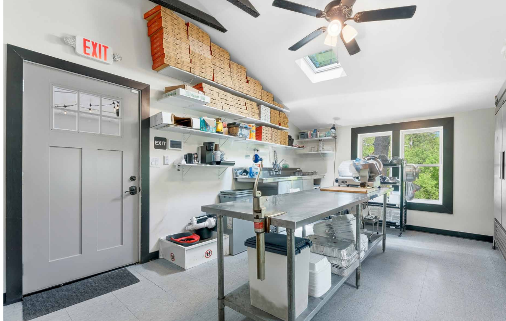
Restaurant Commercial Kitchen.
