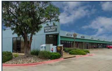
Bldg A 9921 - 9929 Broadway
