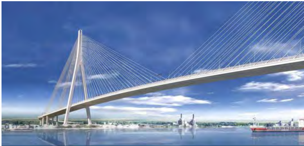
GORDIE HOWE INTERNATIONAL BRIDGE
