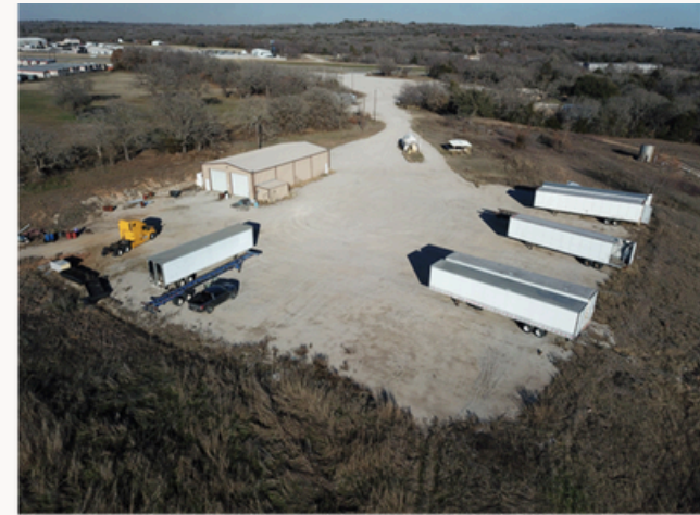
BUILDING 6 AND BACK PARKING YARD
