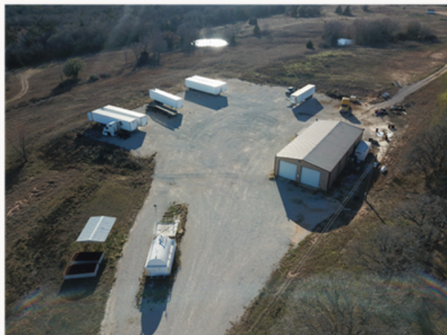
BUILDING 6 AND BACK PARKING YARD
