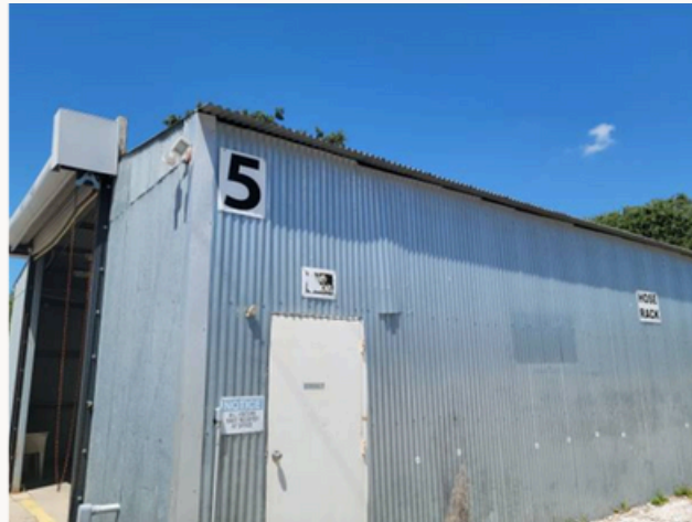
BUILDING 5: SINGLE-BAY METAL
