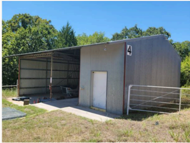
BUILDING 4: METAL STORAGE BUILDING
