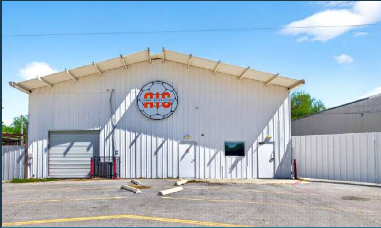
Building A — Front Façade (Fully Air-Conditioned)
