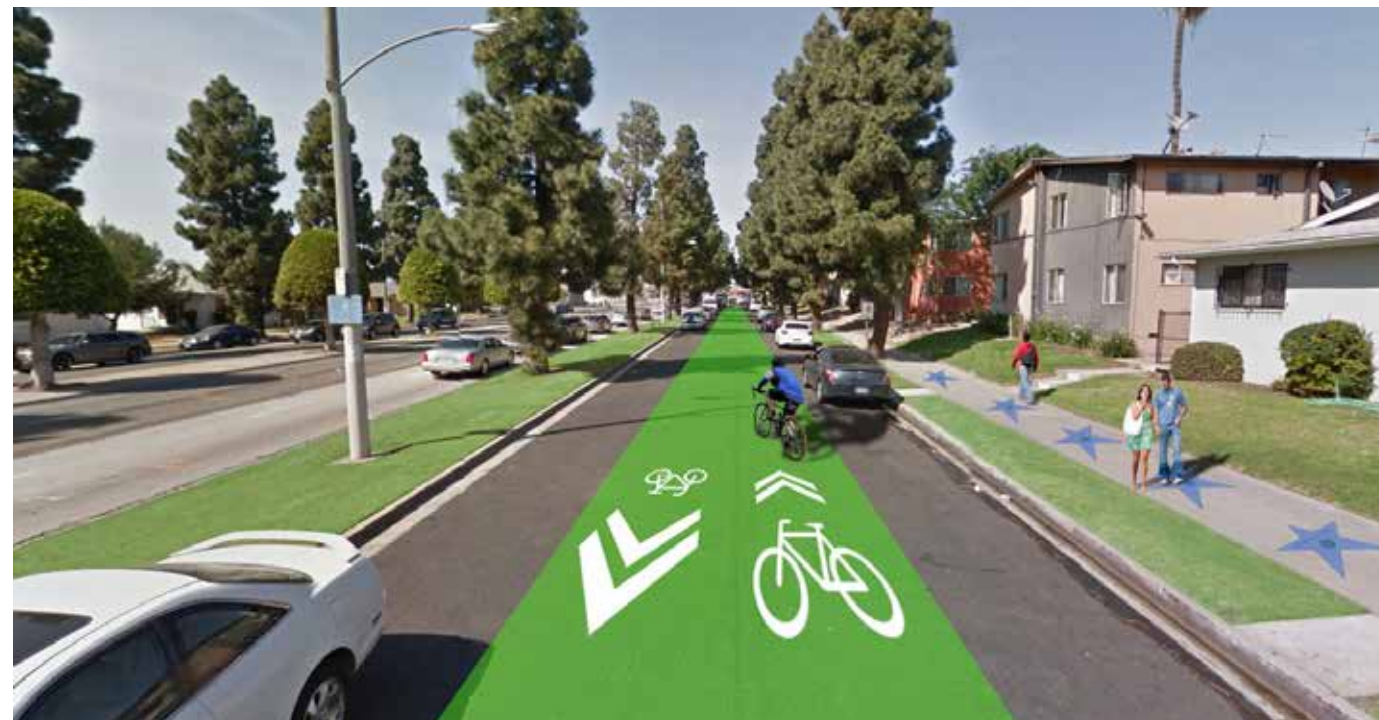
Figure 3.4c Bike sharrows and Champion Mile pedestrian pathway markings added to existing frontage road.
