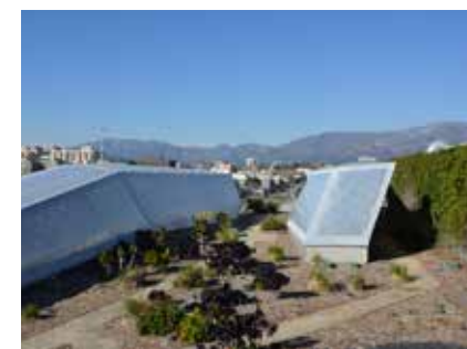
Softscape green roof
