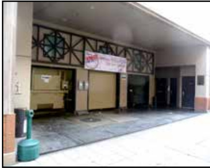
Enclosed trash/loading areas.
