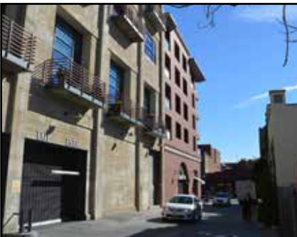
Parking structure access
