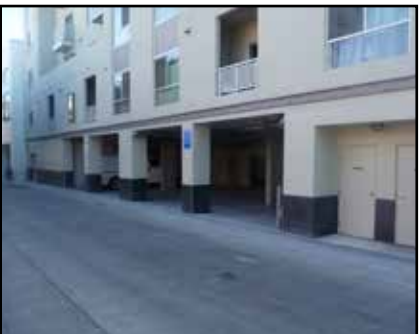
Loading and handicapped parking
