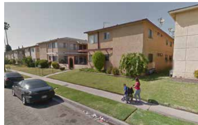
East Gateway Corridor District
