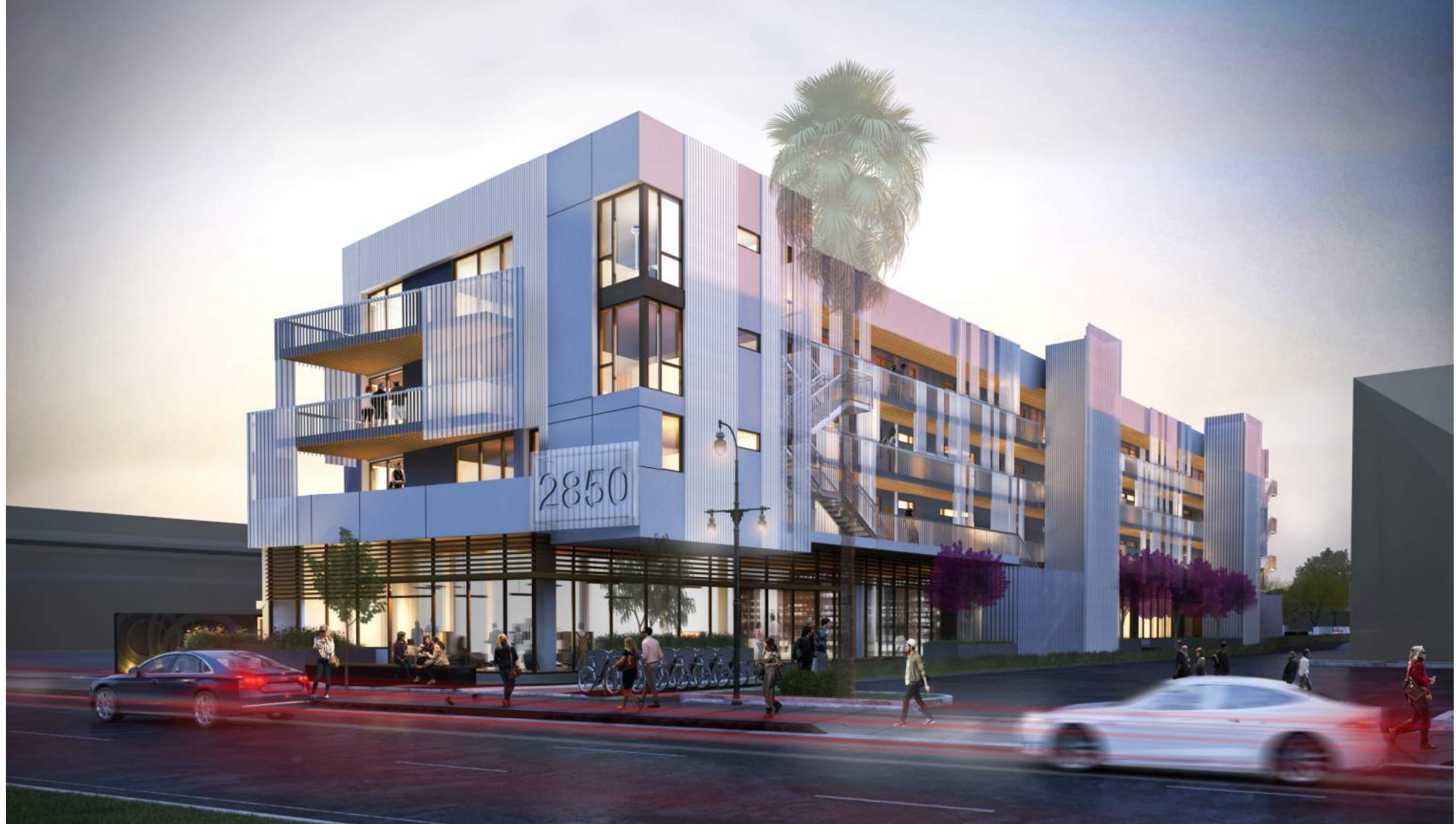
VIEW FROM EL CAMINO REAL LOOKING SOUTH
