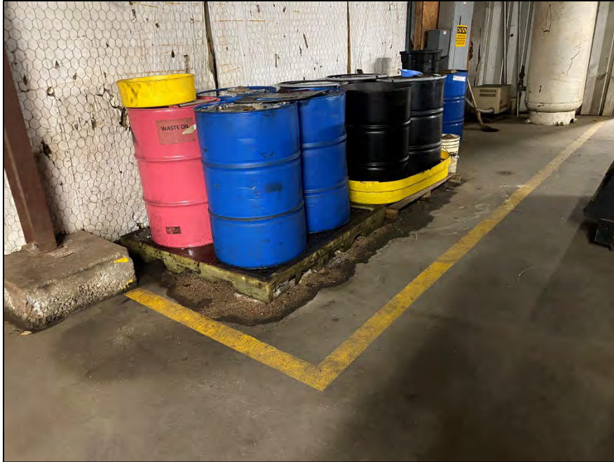
Photo 3. View of pallets where drums of hydraulic oil and used oil are stored. It appears that there are roof leaks that drip in this area and cause the containment pallets to be overtopped by water and the oil floating on top.
