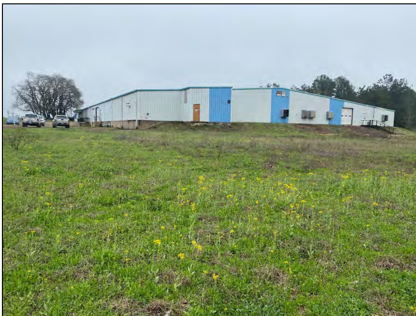
Photo 1. View of exterior of subject property structure from northwest facing southeast.
