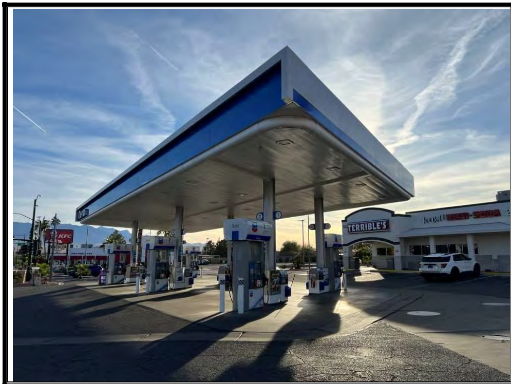
View of Gasoline Canopy of the Convenience Store/Gas Station Component
