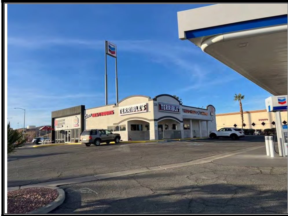
View of Eastern and Southern Elevations of the Convenience Store/Gas Station and Retail Components, Facing Northwest
