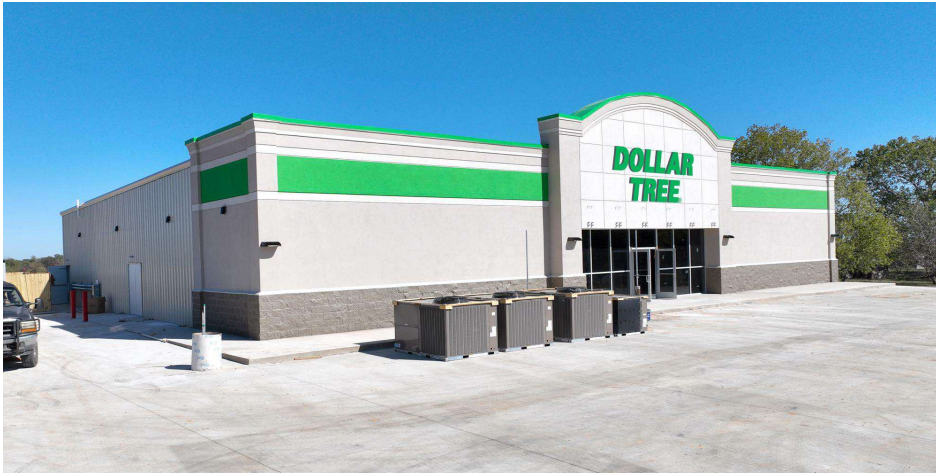
3 Dollar Tree 3320 W Hwy 199 Springtown, TX 76082
